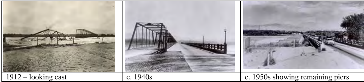
Figure 4: Historic bridge photographs. 1) 1912 after flood; 2) c. 1940s after the concrete bridge was constructed adjacent to the steel truss; and 3) c. 1950s after the steel truss had been removed, but the piers remained in the river.
