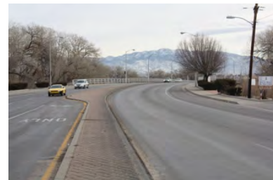
View of Rio Grande bridge (east)
