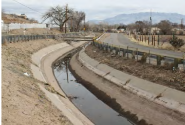
Arenal Main Canal
