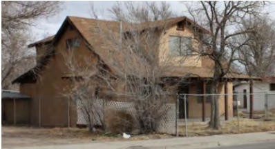
Two story gable house
